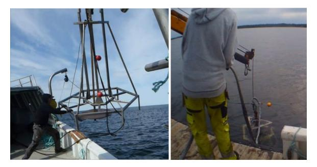
Figure 5. Left: Setting of the 20 helix side-anchors in 2016. It was hard to maneuverer the swinging drill-rig from a classic round-bottomed fishing boat. The original big plates shown in the picture were soon exchanged to smaller plates that could penetrate the sand-bottom. Right: Setting of 27 vertical anchors in 2017. This job was done with part of the rail removed, a new wooden deck, and perfect weather conditions.
