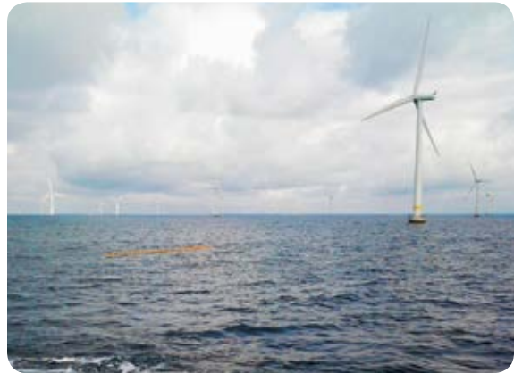
Figure 8: Test cultivation line at Rødsand II: 90 windmills, 207 MW, 75–80 km cables, area of 34 km 2 plus surrounding restricted area.
